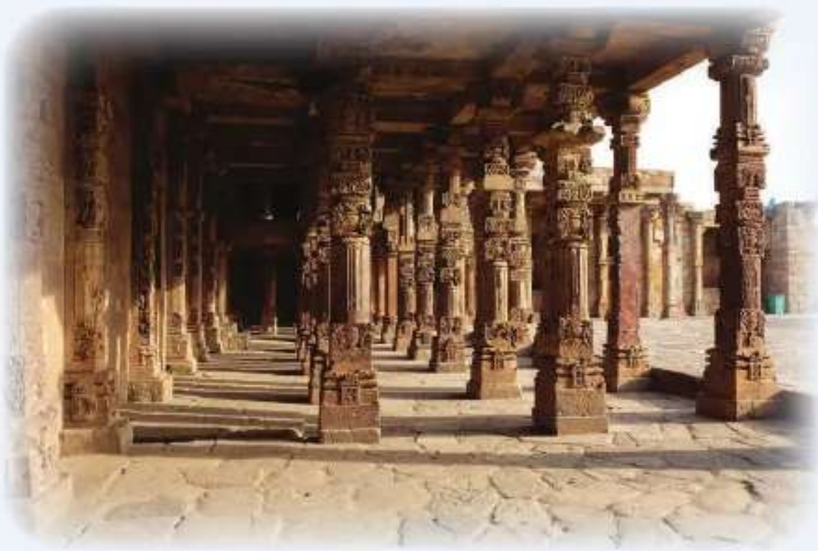
Corner Detail of Qutb Minar complex
