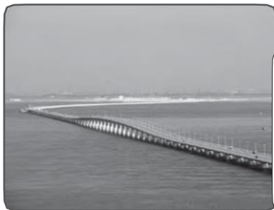
King Fahd Causeway: opened 1986 / actually a series of bridges and dam / 2500 metres long
