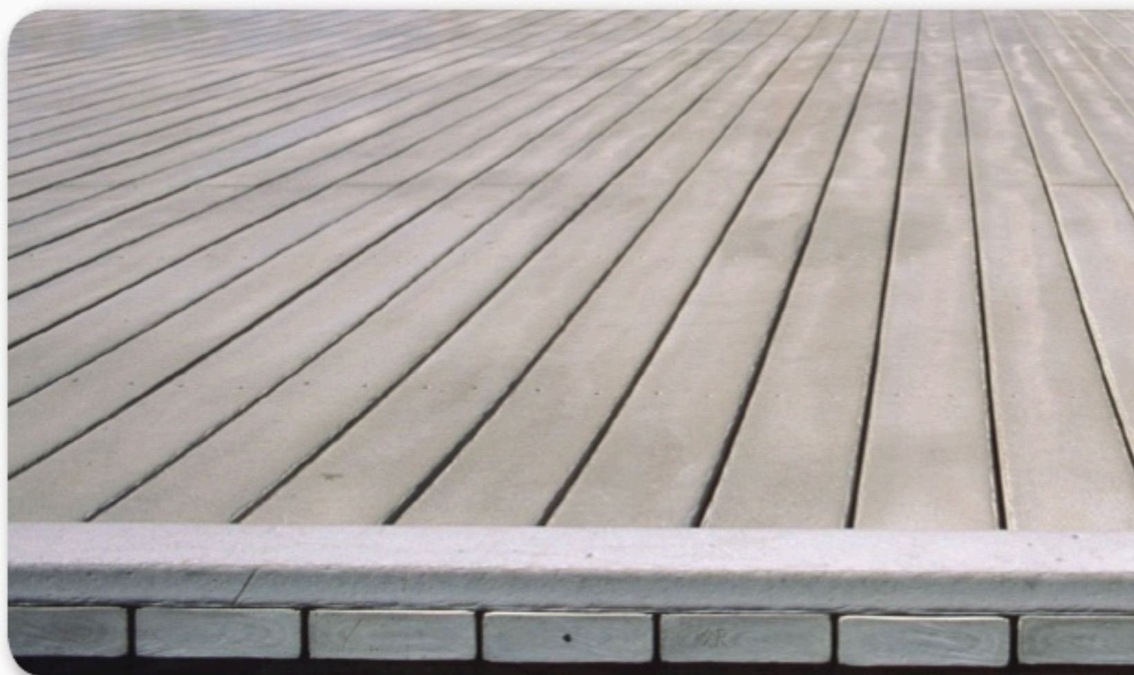
■ Figure 20 Plastic lumber is made from recycled plastic, such as used soft-drink bottles, milk jugs, and other polyethylene waste.
