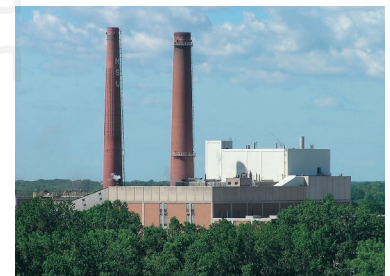
FIGURE 1.19 A coal-fired power plant at Michigan State University that incorporates an electrostatic precipitator to remove particulates from its emissions.
